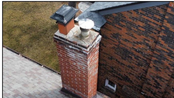
7. Cracked and no drip edge
