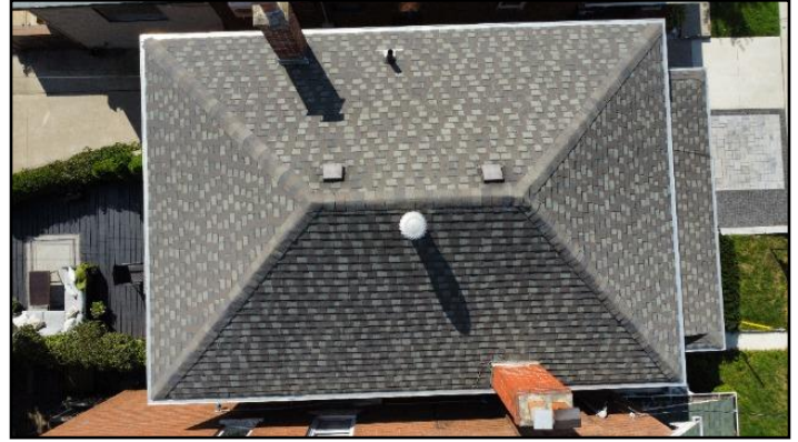
2. Asphalt shingles -- Good condition
