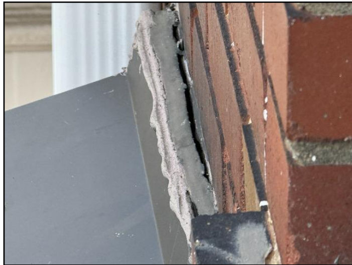
5. Damage, loose, open seams, patched
