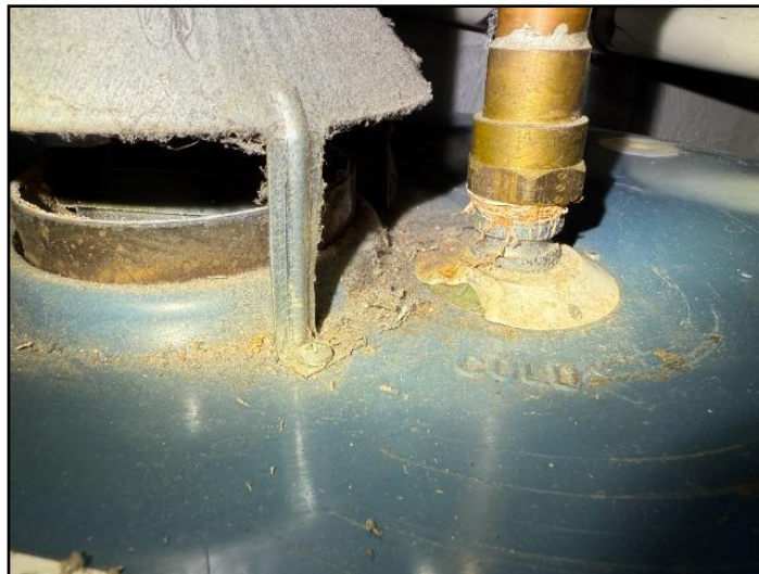
34. Spillage or backdraft at the draft hood
