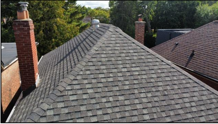
1. Asphalt shingles -- Good condition
