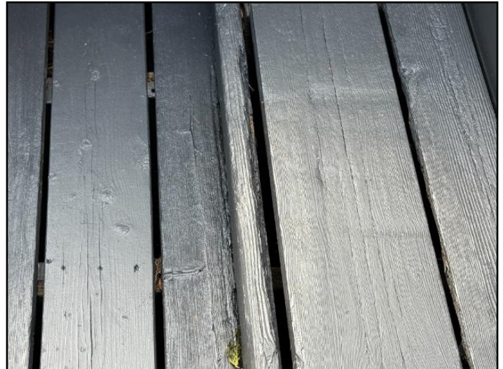
16. vertical board not well secured
