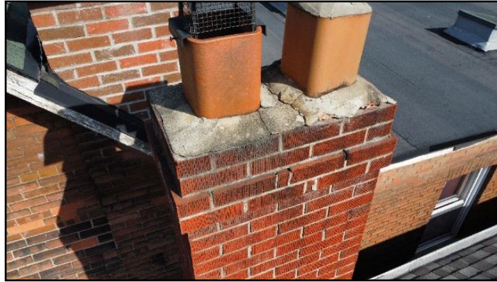
32. No drip edge on cap (crown)
