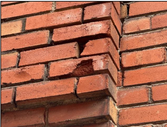
12. example of spalling
