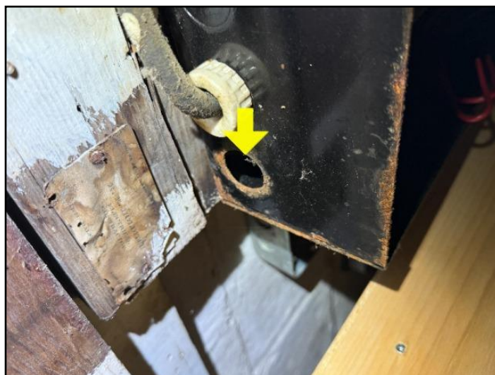
22. Unprotected openings
