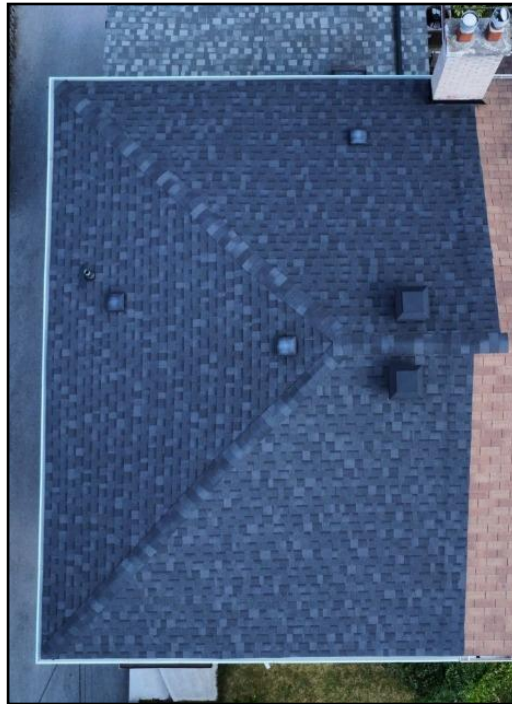
4. Asphalt shingles -- Good condition
