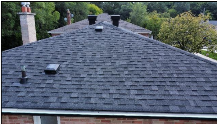
2. Asphalt shingles -- Good condition
