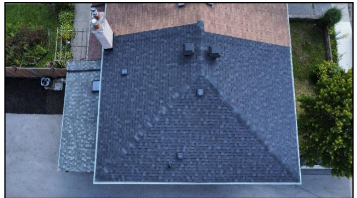
3. Asphalt shingles -- Good condition
