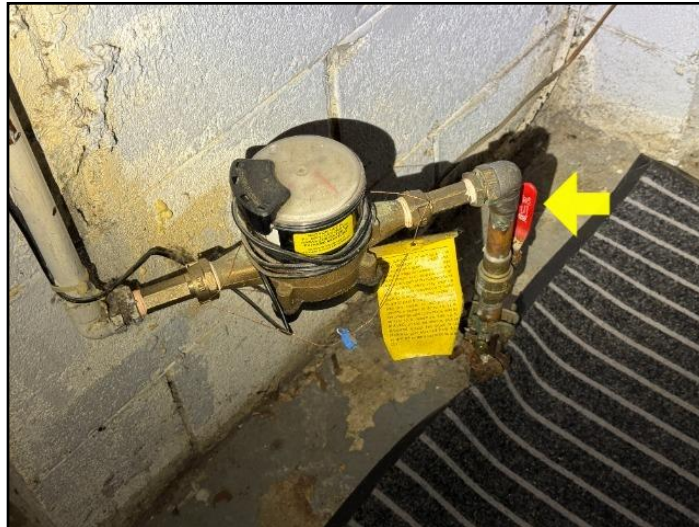
24. Main water shut off valve - Basement
