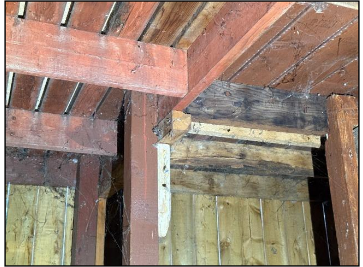
11. example of column/beam supports
