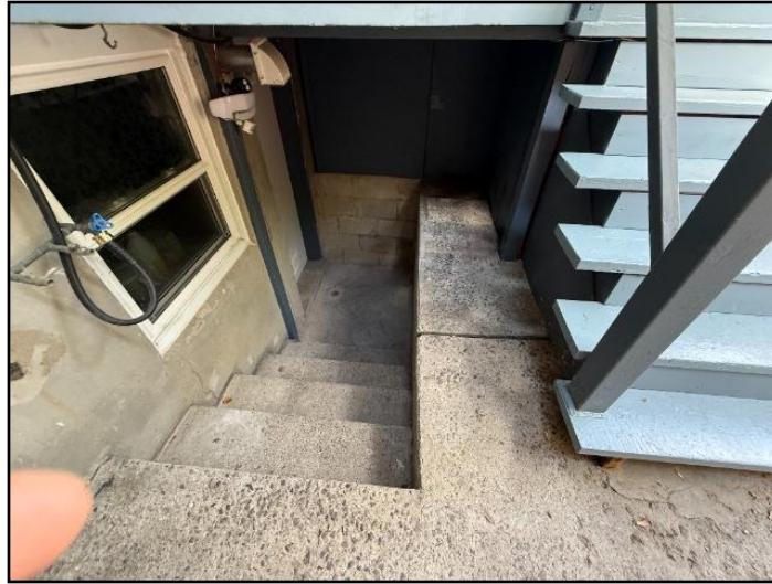
12. Guard and handrail problems
