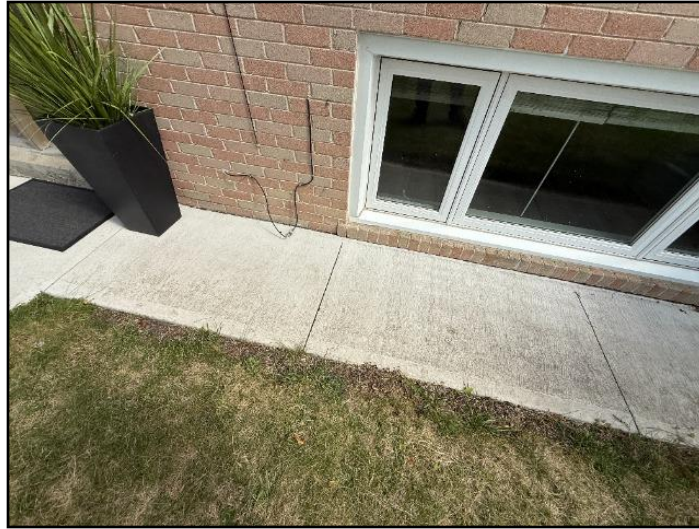
14. Masonry too close to grade
