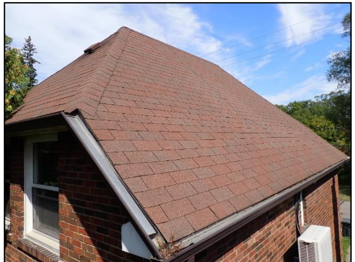
Shingles are in good condition
