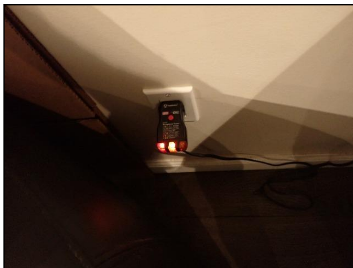
Reversed polarity outlet
