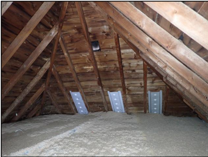
Insulation is evenly distributed
