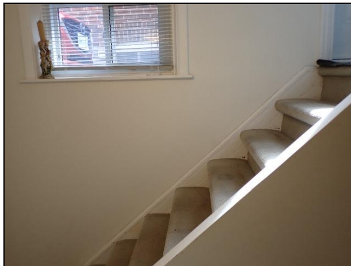
Missing handrail
