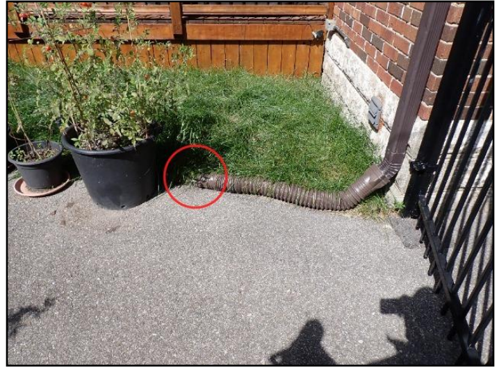
Maintain discharge well away from foundation
