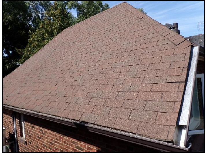
Shingles are in good condition
