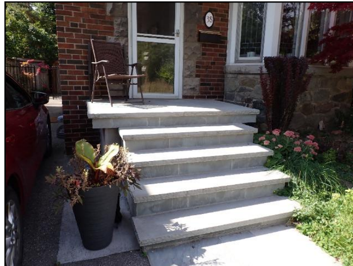
Railings scheduled for installation
