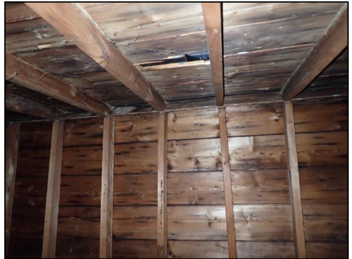
Roof sheathing is clean
