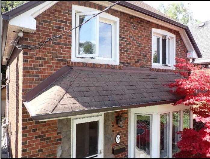
Shingles are in good condition
