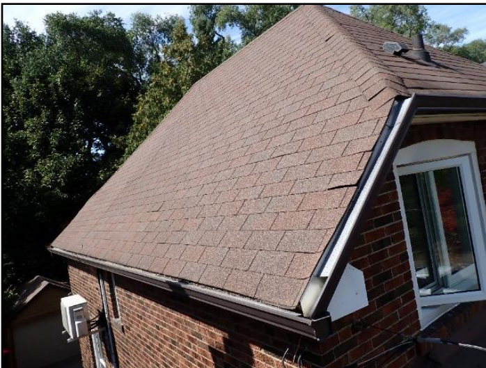
Shingles are in good condition
