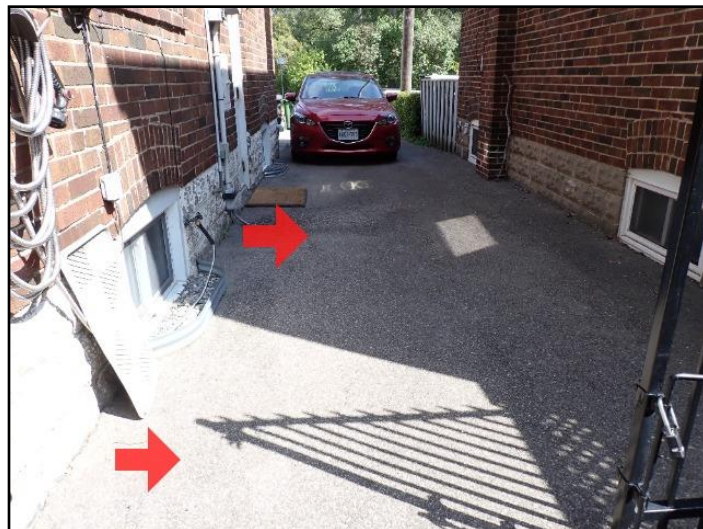
Maintain slope away from house
