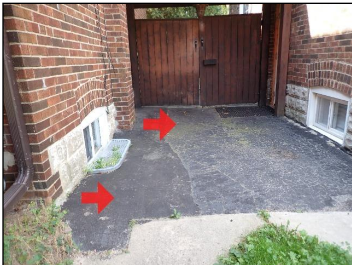
Maintain slope away from house
