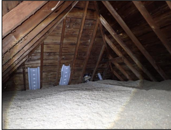
Insulation is evenly distributed
