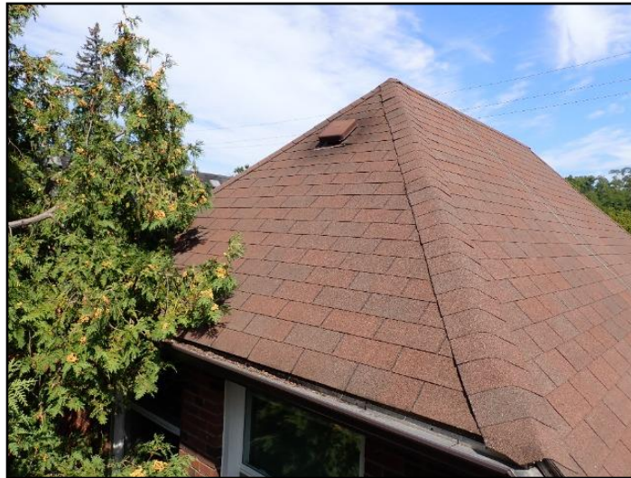
Shingles are in good condition
