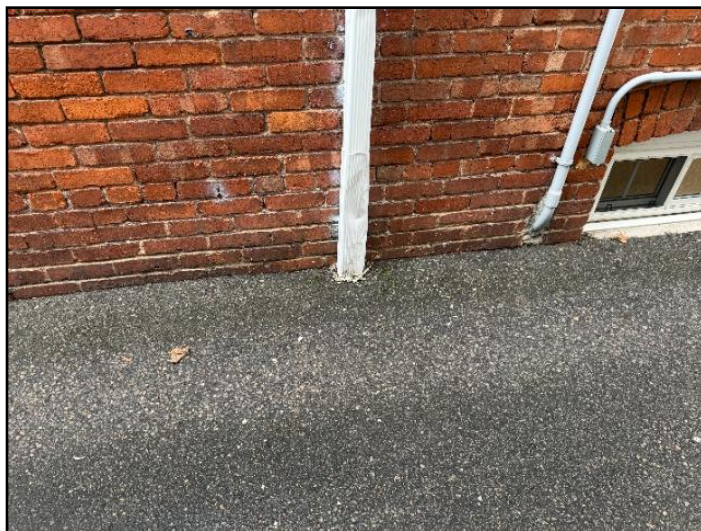
5. Downspout discharge below grade
