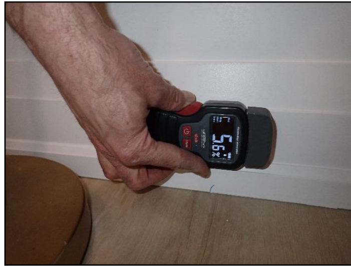
Rear - Typical reading noted - Dry
