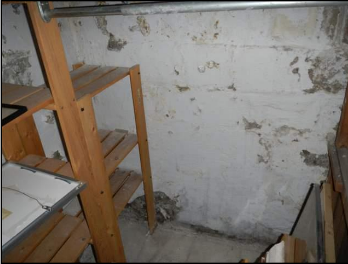
Efflorescence
