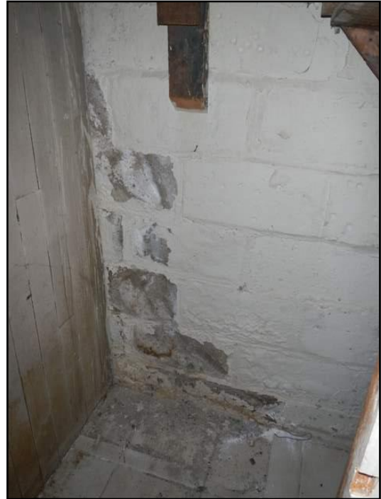
Efflorescence
