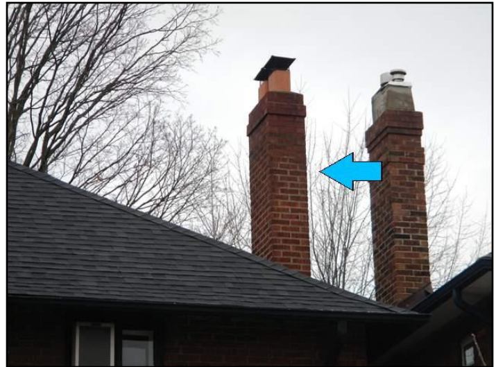
Masonry: rear/right side
