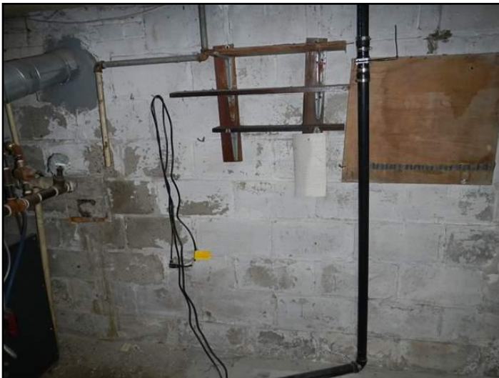
Efflorescence
