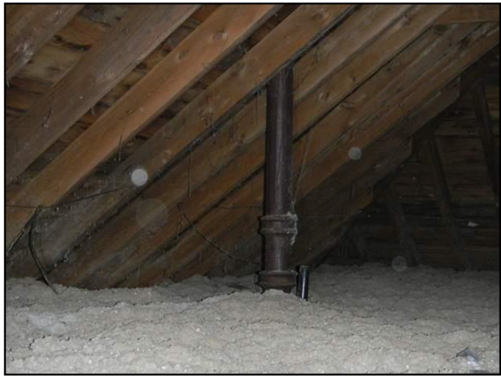
Cast iron in the attic.
