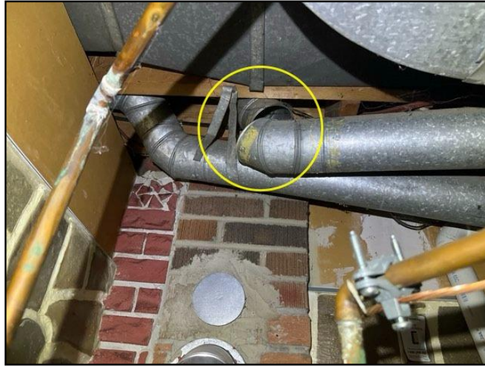
Disconnected ducts
