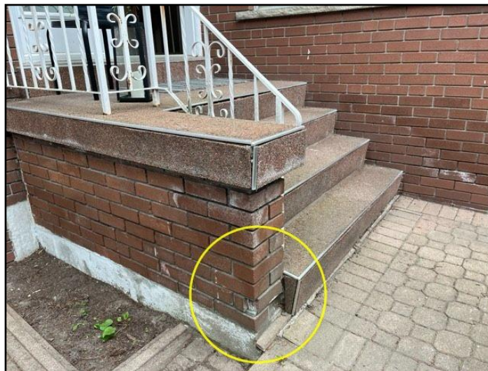
Masonry deterioration
