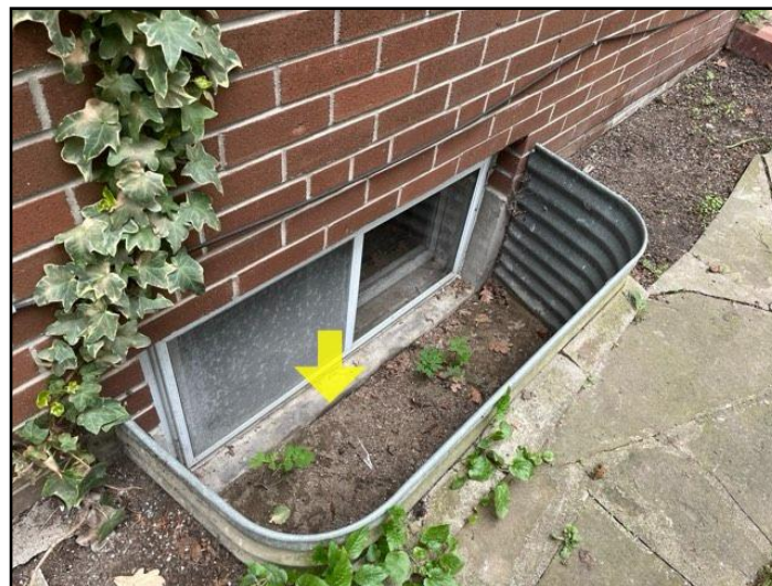
Window close to grade in well
