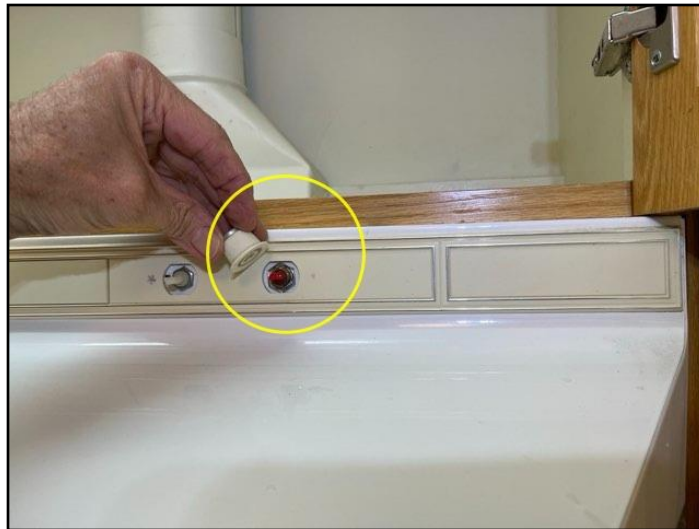
Control damaged
