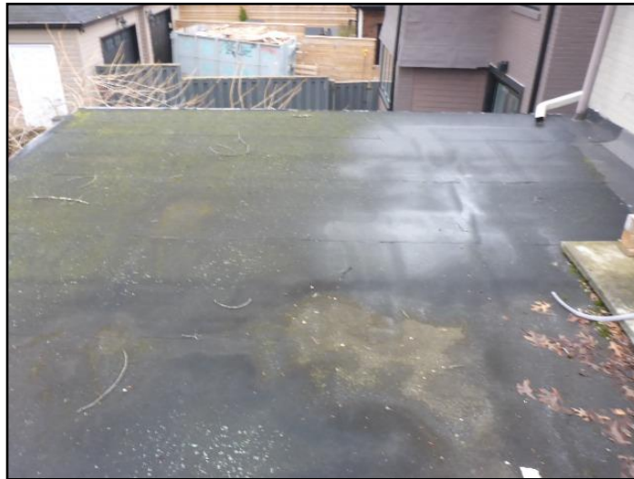
Modified bitumen membrane
