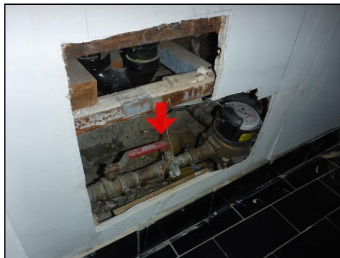
Front of the basement
