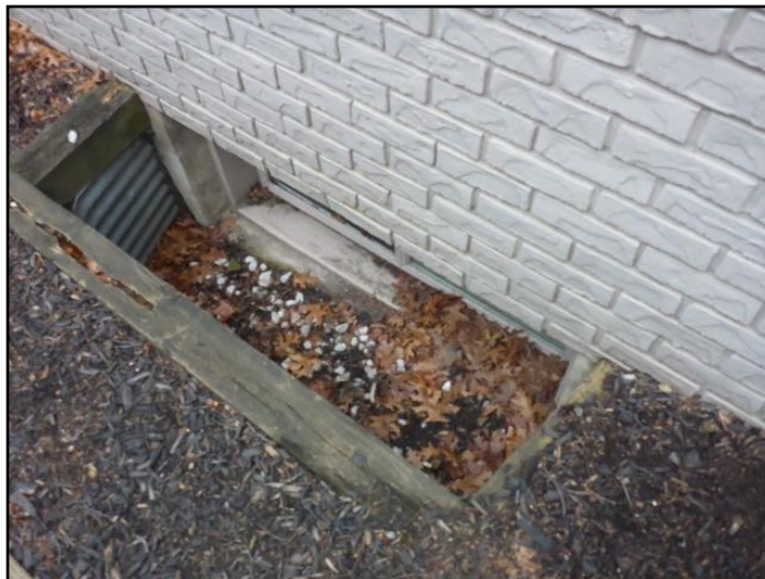
Window close to grade in well
