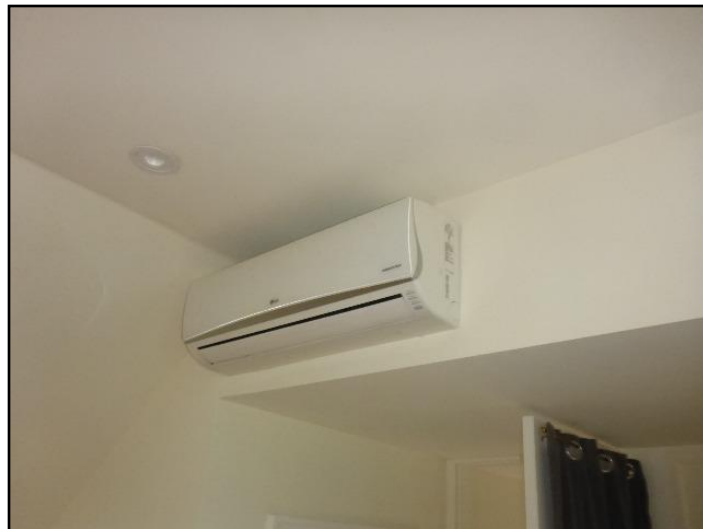
Ductless system- typical indoor unit
