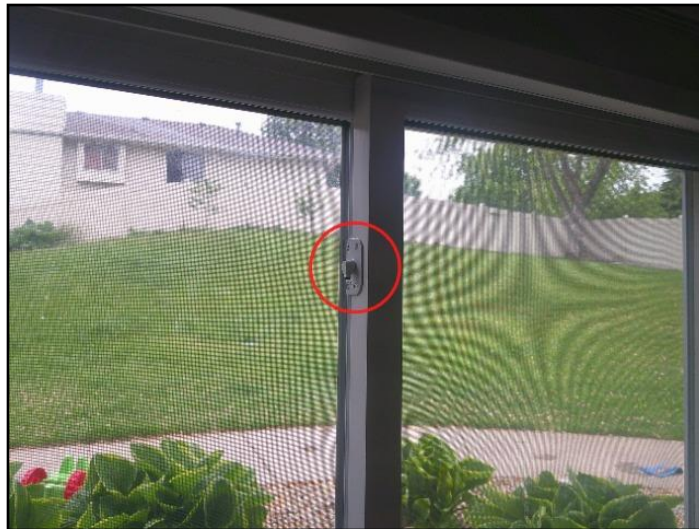
66. Broken lock lever
