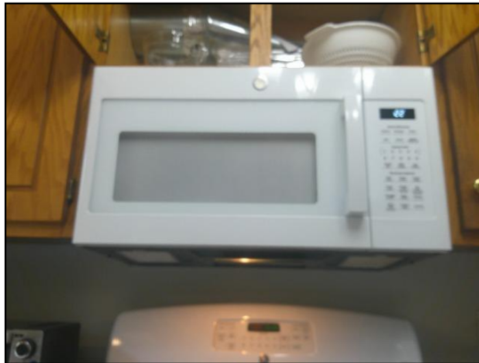
54. GE microwave and exhaust tested
