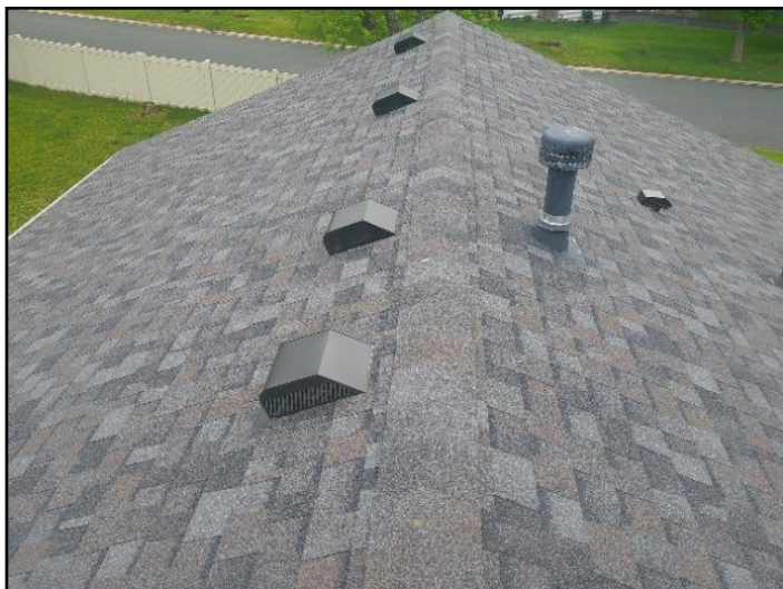
2. Asphalt shingles
