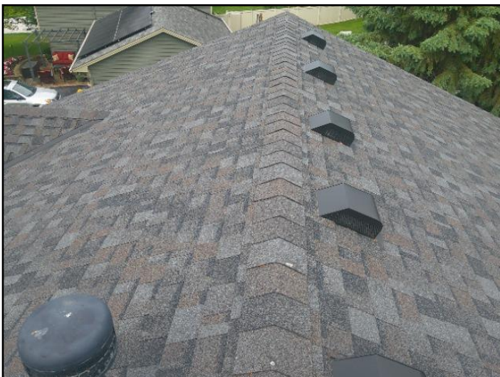
1. Asphalt shingles
