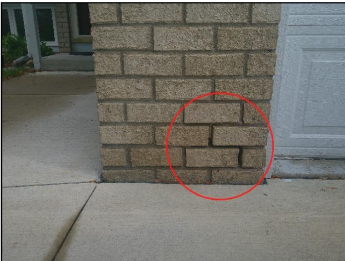
10. Mortar deterioration
