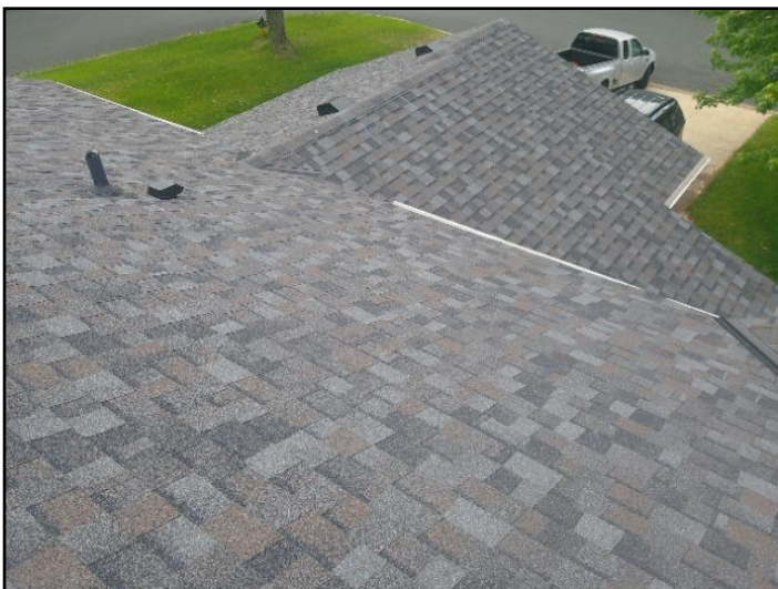
3. Asphalt shingles
