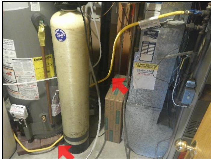
47. Inadequate support
