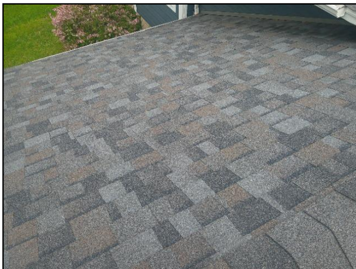
4. Asphalt shingles
