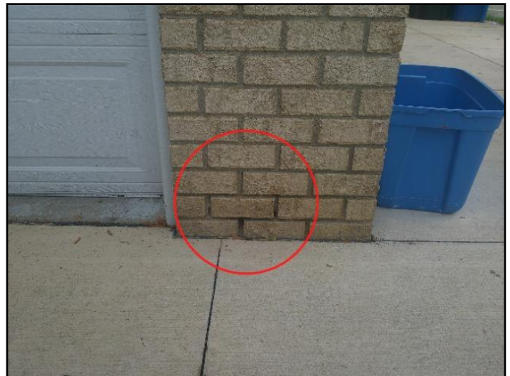
11. Mortar deterioration
