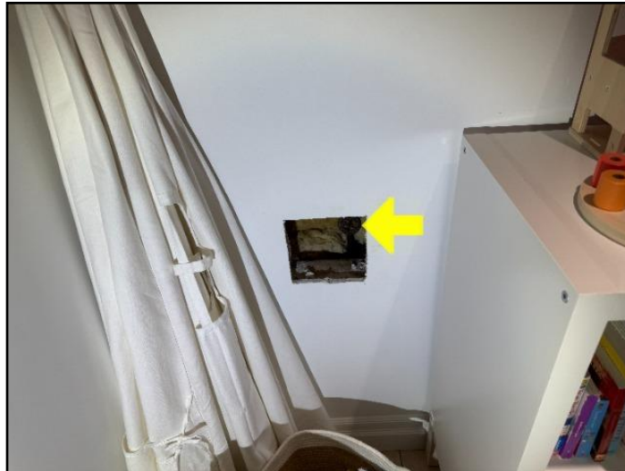
16. Main water shut off valve - Front of the...
