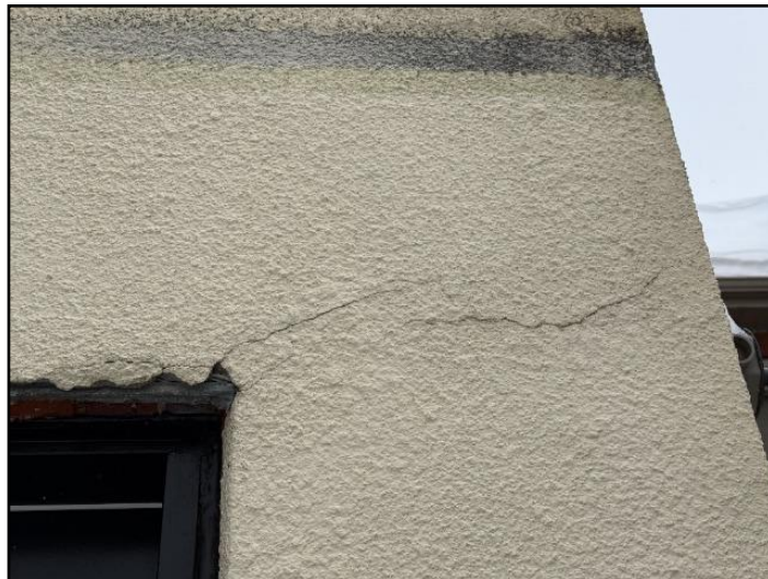
5. Minor cracks example
