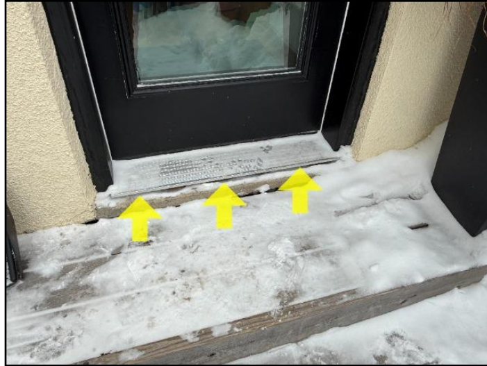
6. Caulking missing, deteriorated or loose
