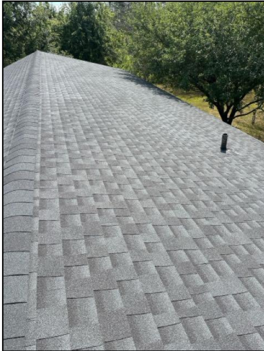
1. Asphalt shingles
