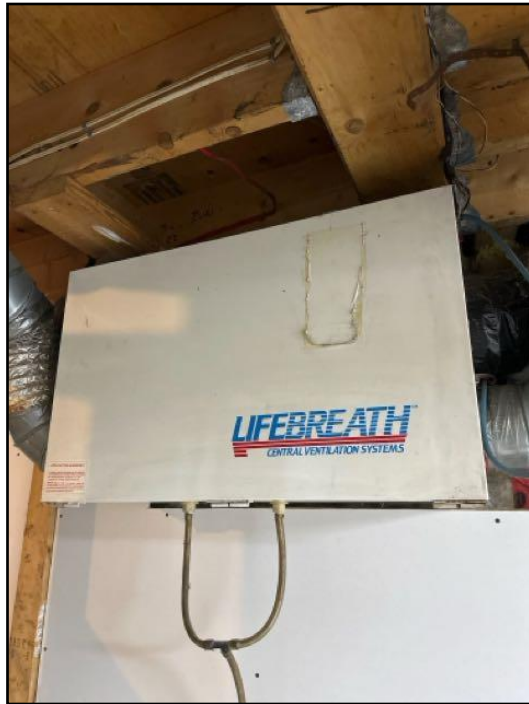
64. Heat recovery ventilator (HRV)
