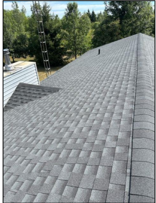
2. Asphalt shingles
