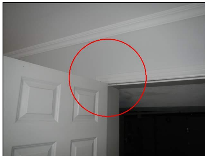
Door closer - missing
