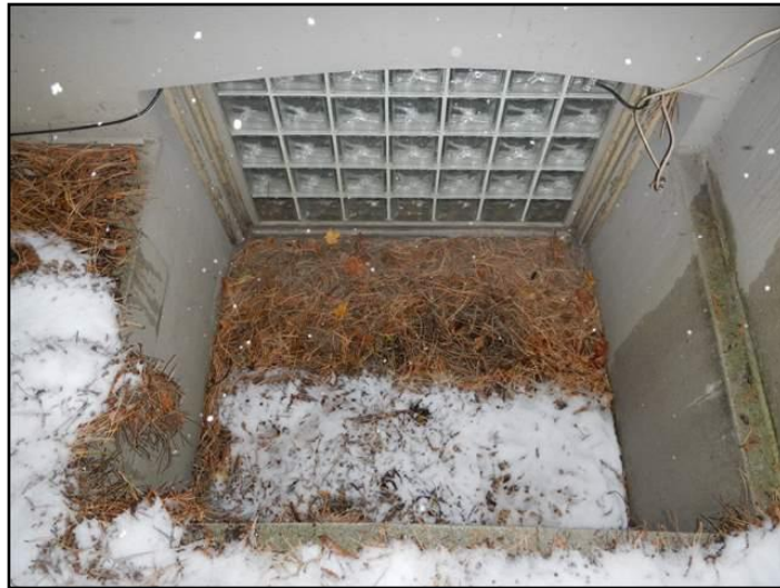
Window close to grade in well
