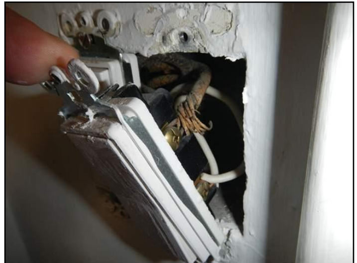
Copper - knob and tube
