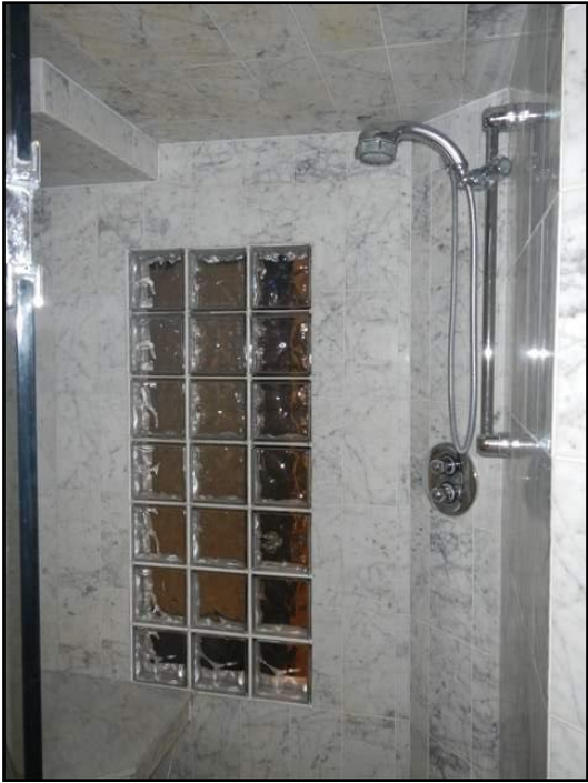
Shower - Window vulnerable -
