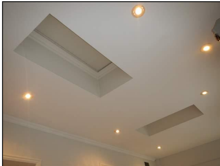
Skylight(s) - vulnerable area -
