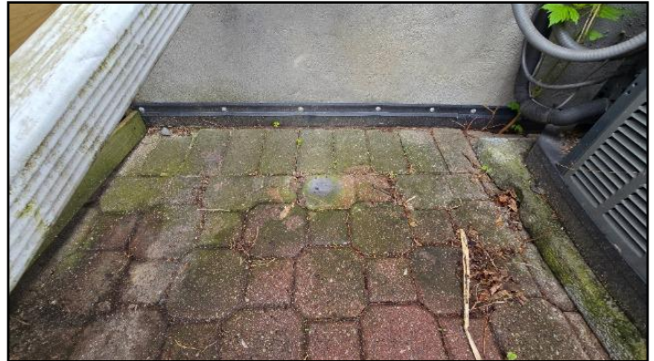
32. Water proofing was added to the homes...
