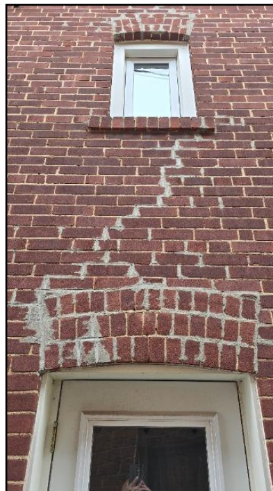
7. Mortar deterioration
