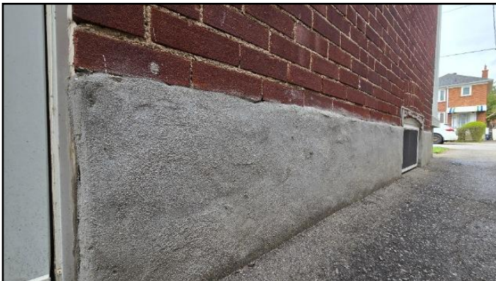
28. Parging noted at foundation walls
