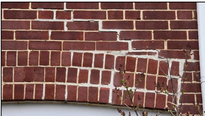
6. Mortar deterioration
