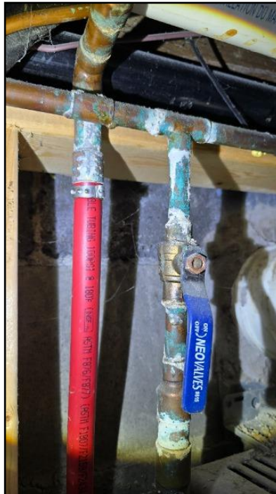
89. Corrosion Noted
