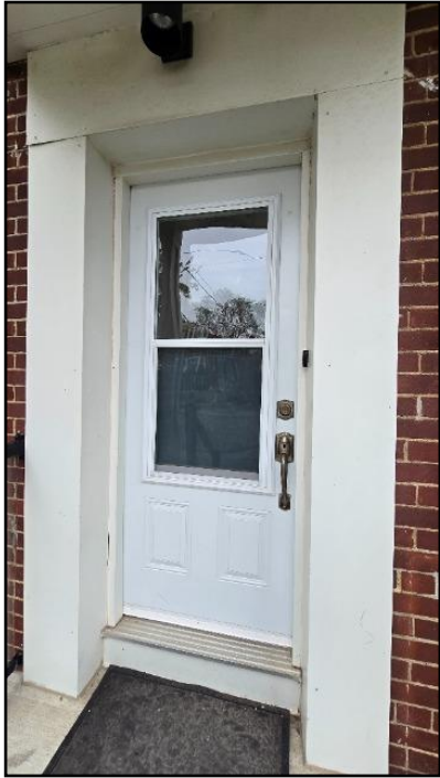
114. Various Doors Noted
