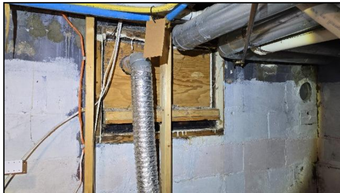
9. Original window removed
