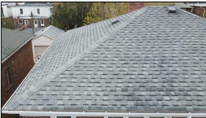
2. Asphalt shingles
