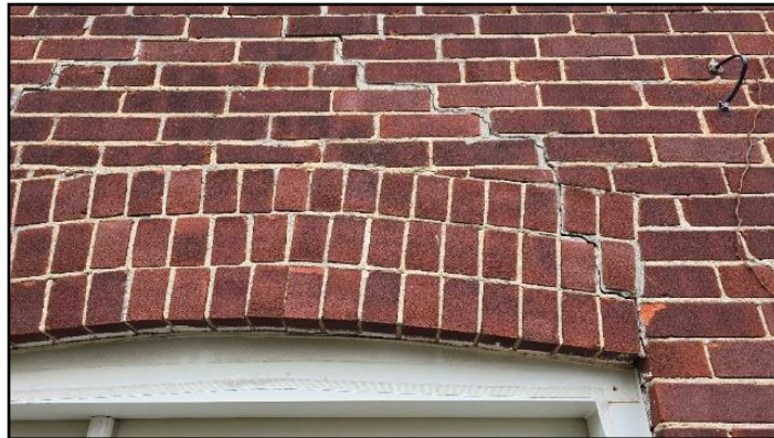
8. Mortar deterioration
