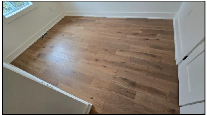
110. Various flooring noted
