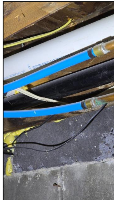
92. PEX (cross-linked Polyethylene)
