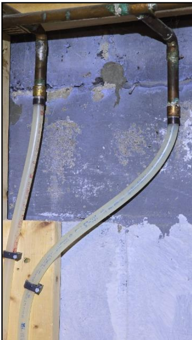
91. PEX (cross-linked Polyethylene)
