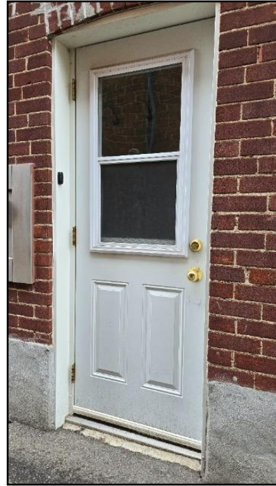
115. Various Doors Noted
