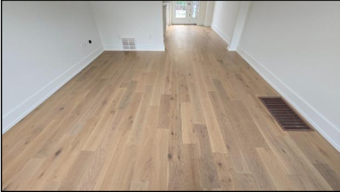
107. Various flooring noted
