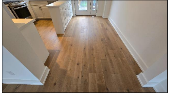
108. Various flooring noted
