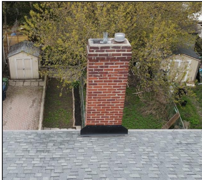
77. Interiors of vent systems, flues, and...
