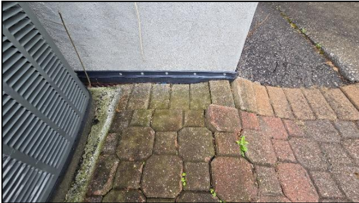
31. Water proofing was added to the homes...
