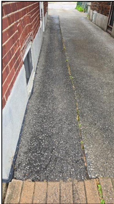
33. Water proofing was added to the homes...
