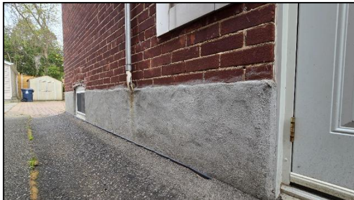
29. Parging noted at foundation walls
