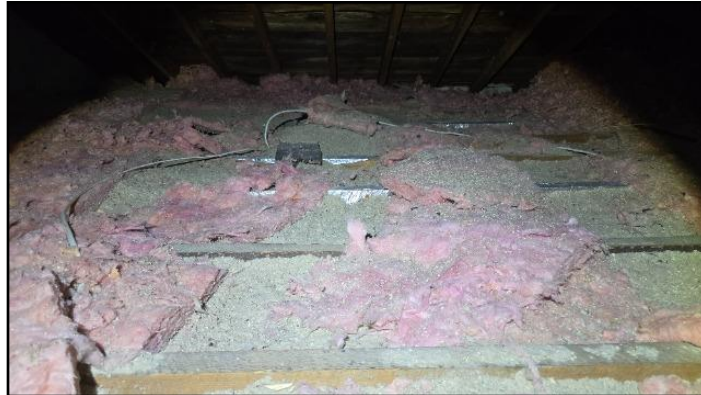
86. Fiber Glass/Cellulose Combination
