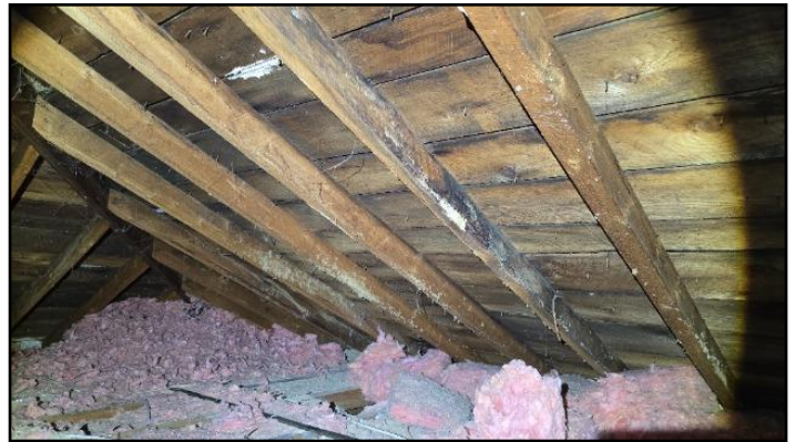
37. Rrafters/ceiling joists
