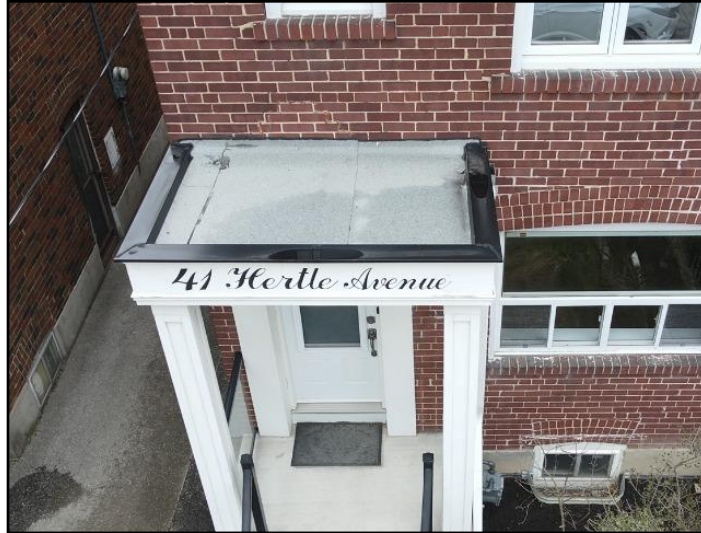
4. Modified bitumen membrane
