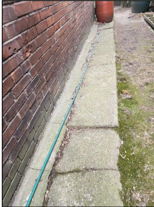
7. Improper slope or drainage
