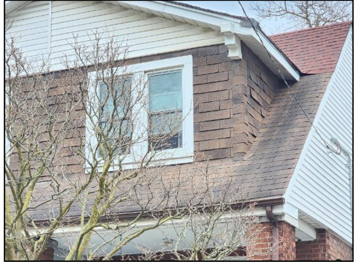
2. Asphalt shingles
