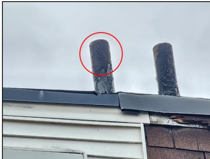
20. Cast iron drain pipes. (Past its typical...
