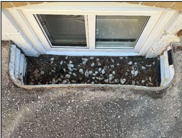
4. Less than 6 inches below window
