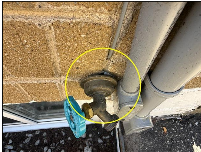
22. Handle loose OR damaged
