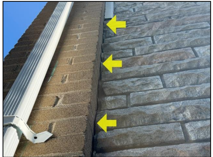
14. Mortar missing
