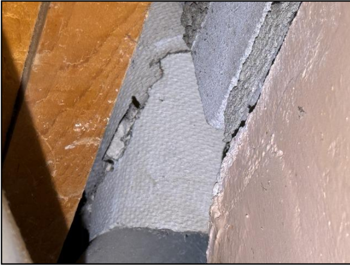
17. Insulation on ductwork may contain asbestos
