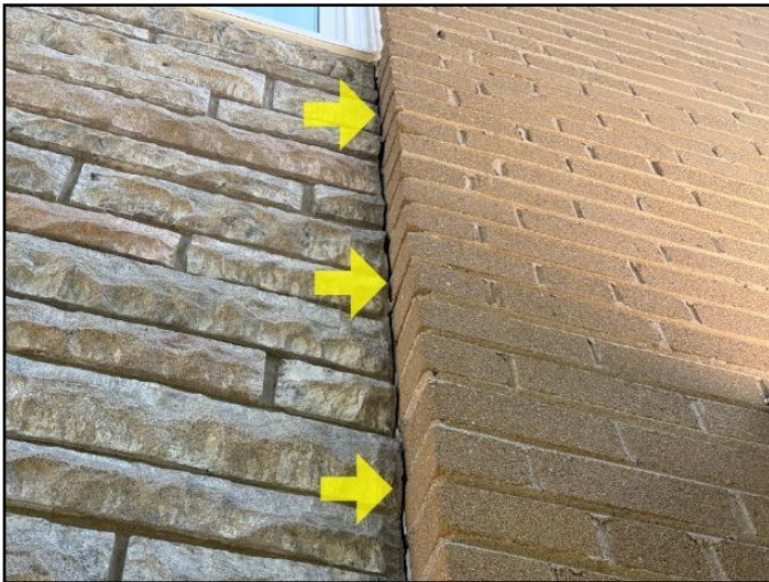
13. Mortar missing
