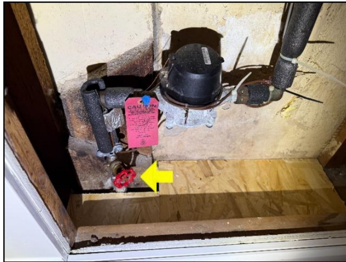
21. Main water shut off valve - Basement
