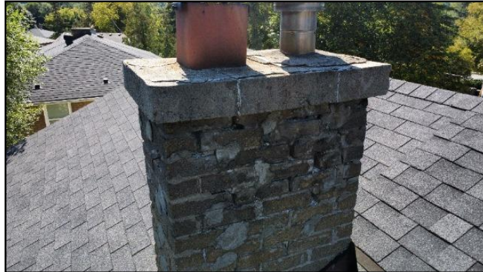
19. Loose, missing or deteriorated masonry...
