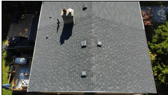
1. Asphalt shingles -- Good condition
