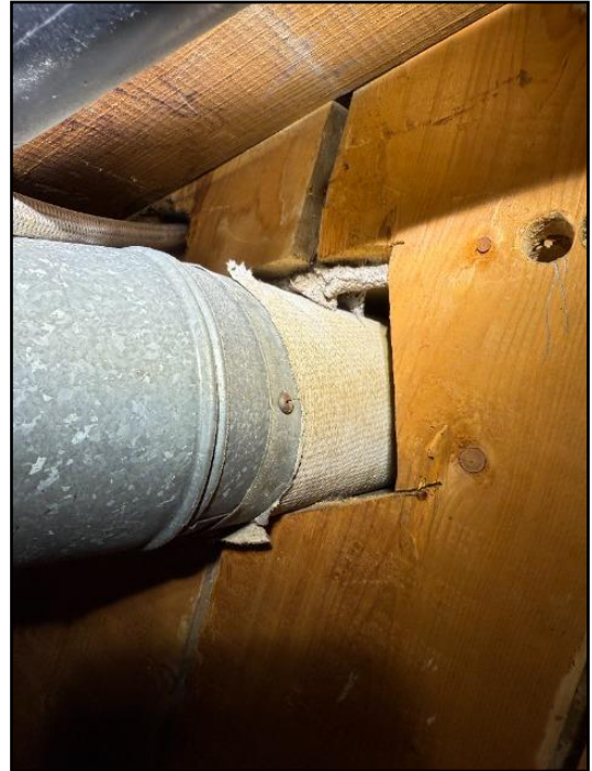
18. Insulation on ductwork may contain asbestos
